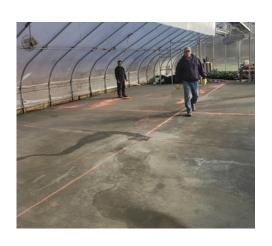
The Lakeview FFA greenhouse has recently been undergoing tremendous renovations. The front three-fourths of the floor are now cement with two drains installed, and plans are underway to make an in-ground planting area in the back. The roof was also recently replaced and has made a great difference already. The grow towers and aquaponics system are now up and running and should be providing fresh produce soon.
